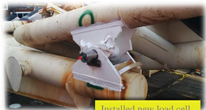
Installed new load cell
