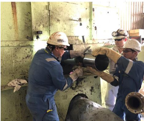
Installing of sleeve
